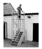
When working at platform heights of 2mts. and over (9 rungs from the base) the tower should be stabilised, tied in, or braced against the building.
